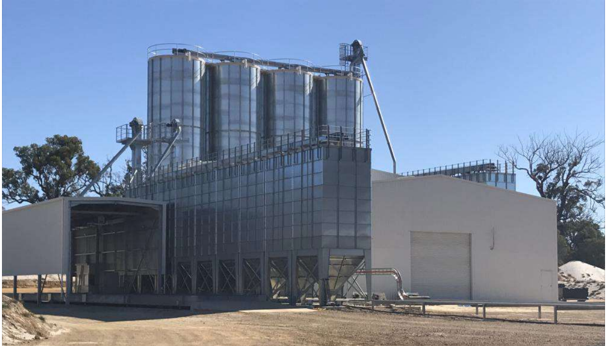
Figure 5: Photo of the feed mill facility in place at Westpork Kojunup. The facility is proposed to be relocated to Glenlevit Piggery.
