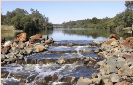
Taken when it was first installed, looking upstream
