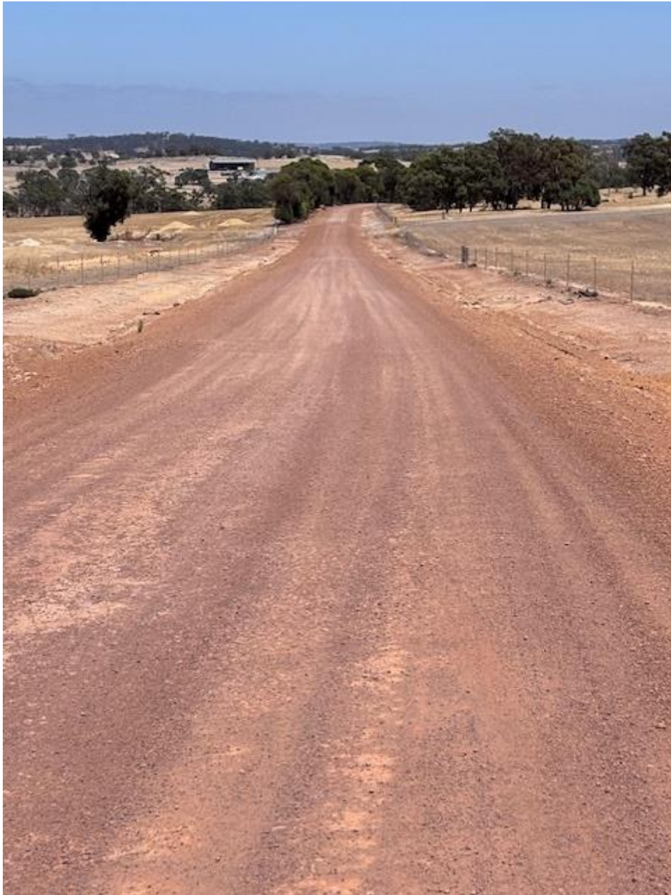
Popanyinning East Road gravel sheeting
