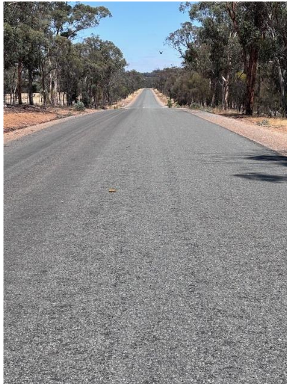
Cuballing East Road – final seal (WSFN)
