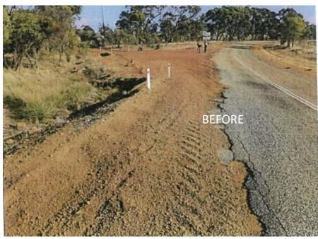
earth works installed. In year two the road was built to level, the intersections with Nebrikinning and Springhill Roads were constructed and the final seal provided.
