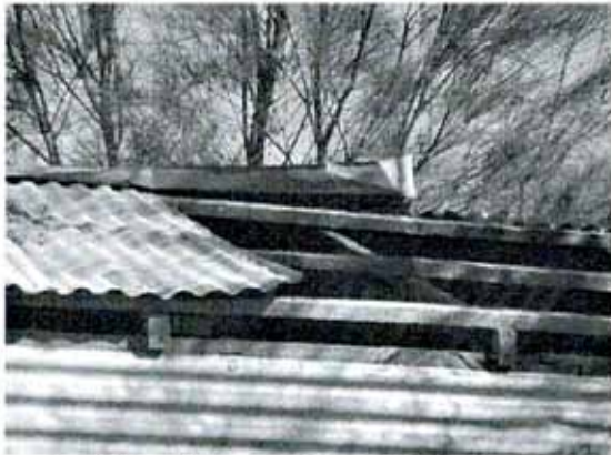
Shearing Sheds and Old Machinery Sheds Roof Re-Screwing
