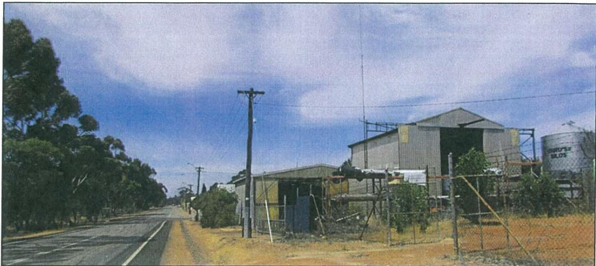
Photograph 1 – View of subject site looking south along Francis Street.
