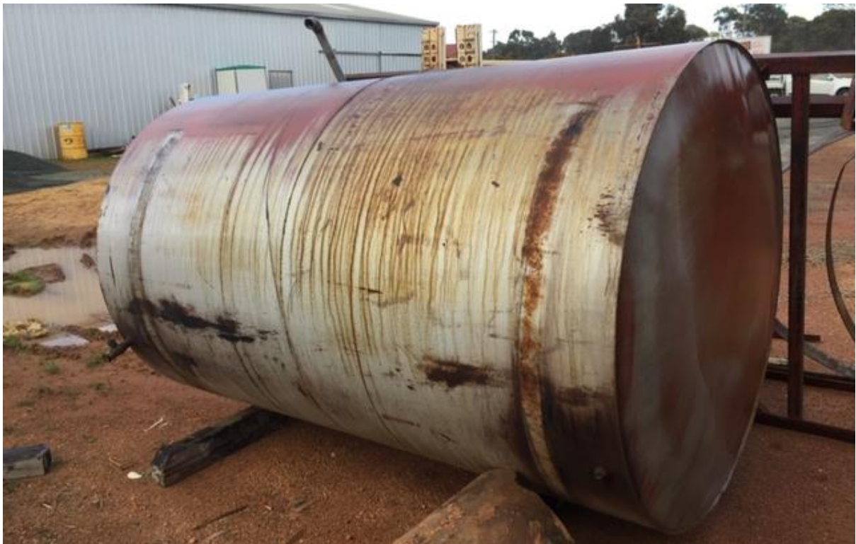
4,000 litre diesel tank and frame
